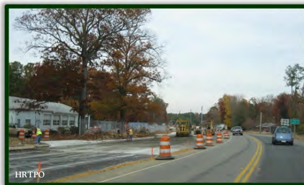
Ironbound Road Construction
