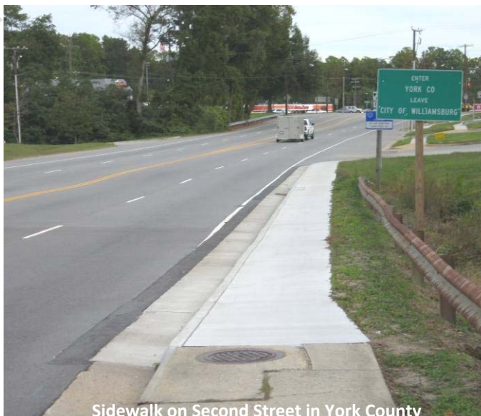
Sidewalk on Second Street in York County
